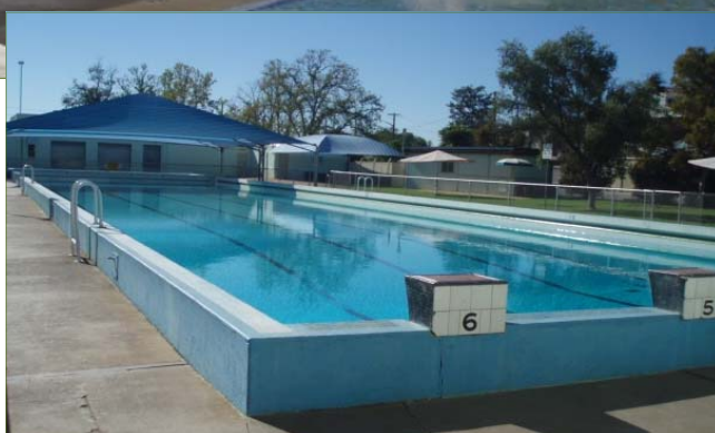
The Forbes Pool. Before (above) and after (top)
