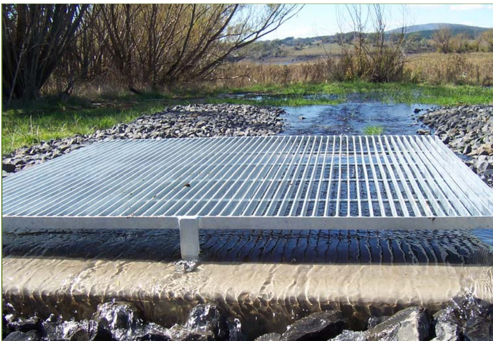
The stormwater harvesting outlet at the edge of Suma Park Dam
